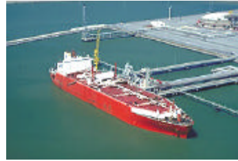
LNG tanker discharging at the Zeebrugge terminal, Belgium. Photo from Fluxys
