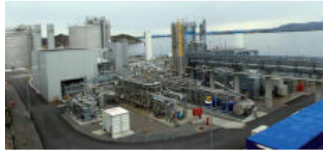
Small scale LNG: Gasnor's LNG plant at Kollsnes, Norway (120.000 tonnes/year capacity)
